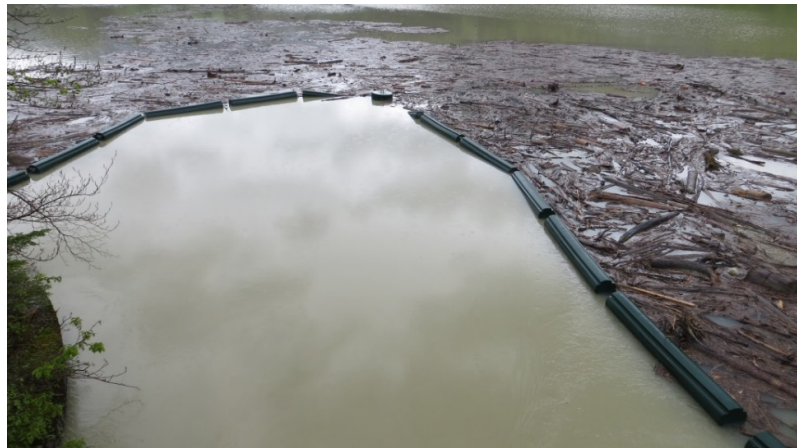
Figure 4: Situation before the floating barrier breach of May 2015
