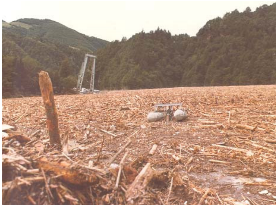
Figure 4: Large wood deposition in reservoir after the 1978 flood event (Source: Ofima)
