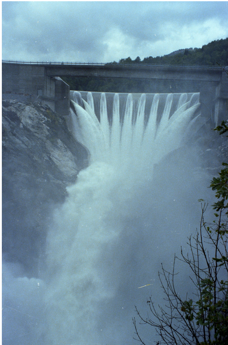
Figure 6: New dam spillway in operation (Source: Ofima)
