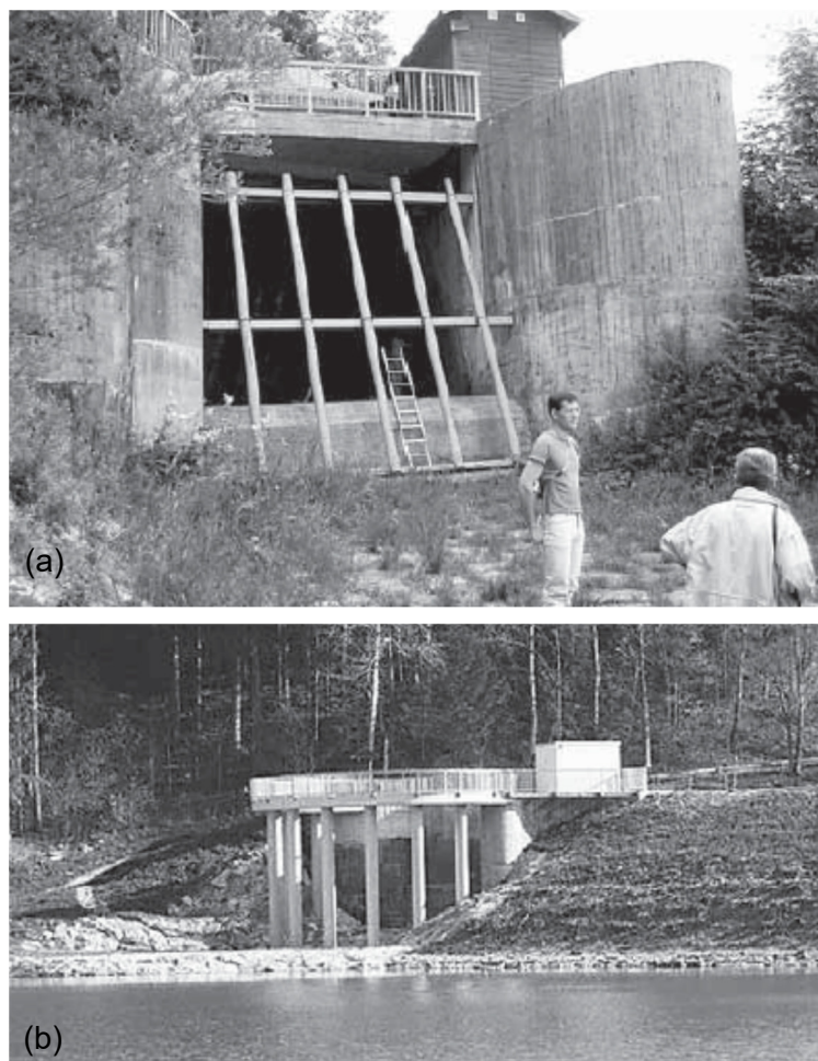
Figure 31: a) Old spillway with large wood rack at Grüntensee and b) new upstream rack pillars (Photo: Hartlieb 2015).
