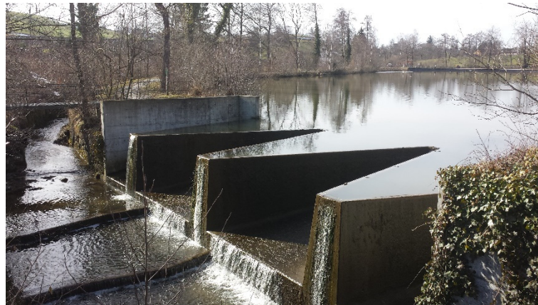
Figure 25: Spillway inlet structure in the form of a labyrinth weir with a large overflow crest and clearance width at Sternenweiher (Canton of Zurich, Switzerland) (Photo: Boes, 2015).
