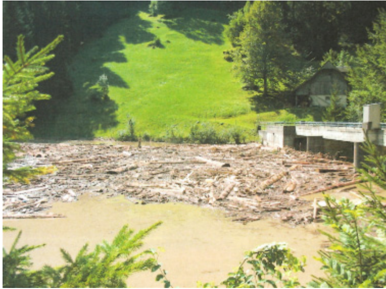
Figure 2: Dam spillway obstruction due to large wood during the 2005 flood (Source: EW Nidwalden)
