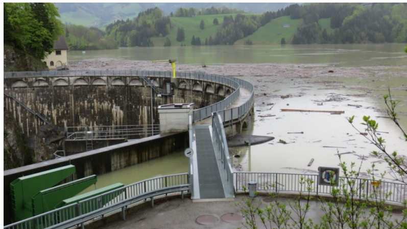
Figure 5: Large wood volumes at Montsalvens reservoir during a flood
