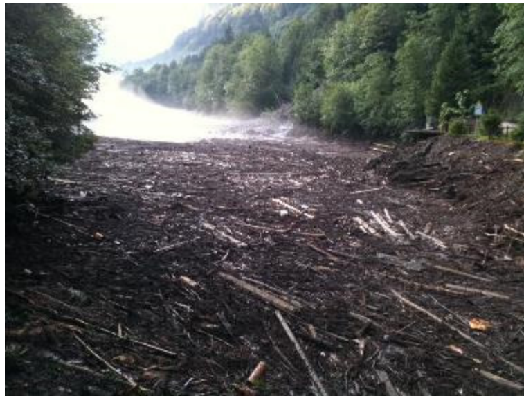
Figure 4: Large wood carpet in the Schlattli reservoir after the 2010 flood event (Source: ebs Energie AG)
