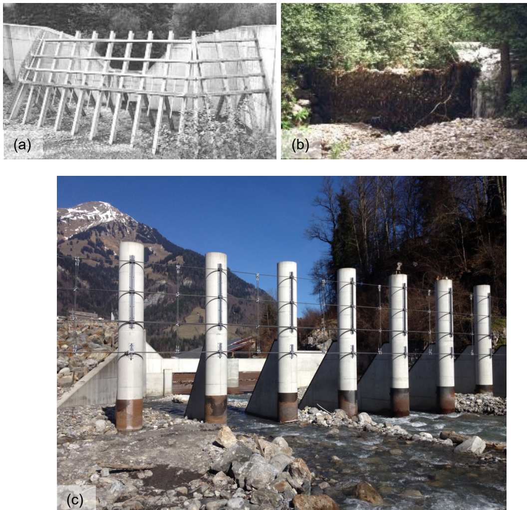
Figure 9: Large wood retention by means of (a) trash rack at the retention basin in Sachseln, canton Obwalden (photo: VAW), (b) cable net at Faukengraben, Upper Bavaria, Germany (photo: Institute for Hydraulic Engineering and Water Resources Management, TU Munich) and (c) Combination of large wood and trash cable racks on the Chiene river, Canton Bern (Photo: Emch + Berger AG).
