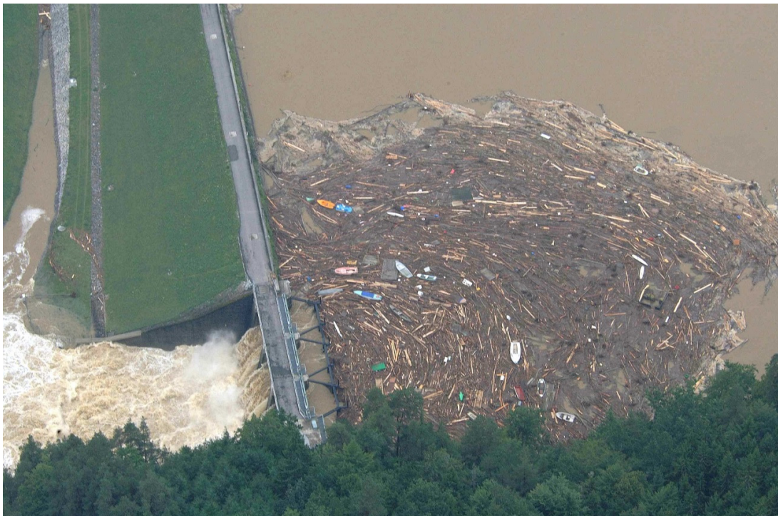
Figure 2: Floating debris in front of the Thurnberg dam spillway on the Kamp river in lower Austria during the extreme flood in 2002 (Photo: Federal Office for Agriculture and Forestry, Environment and Water Management, Austria).
