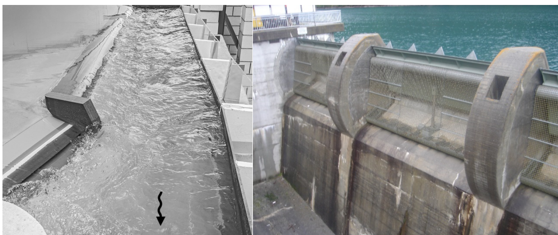
Figure 24: Flood spillway inlet structure in a collecting channel with flaps. Left: top view of a dam spillway model of the Trängslet Dam in Sweden with single-bay flap gate at the downstream side of the weir (Lucas et al. 2015); right: multiple-bay weir with flap gates and flow disturber at the Punt dal Gall dam (Photo: Boes, 2009).
