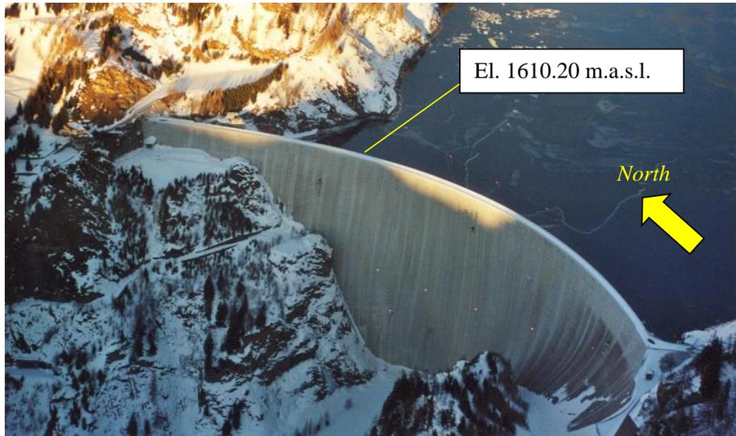
Figure 1 : Luzzone Dam (Switzerland), H = 225 m
