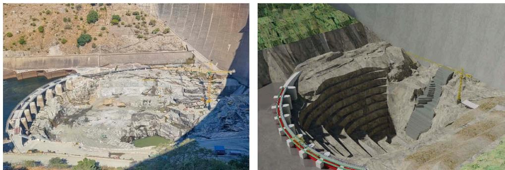
Figure 7. Kariba Dam, Zambia/Zimbabwe - View of the plunge pool (March 2023) and computer-generated view of the reshaped excavation (Razel Bec, 2016).
