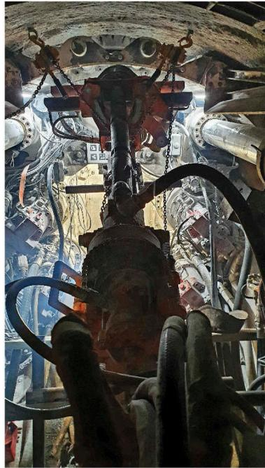
Figure 7. Destruction boreholes by hand behind the cutter head.
