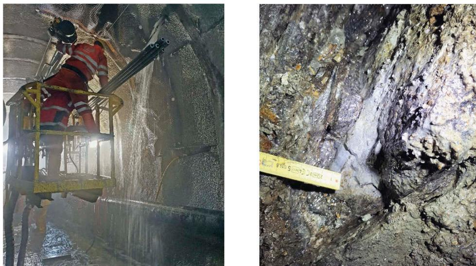
Figure 1. New headrace tunnel excavated at Ritom HPP. (Left) Water inflow. (Right) Discontinuities in the rock efficiently sealed with the hybrid grout.
