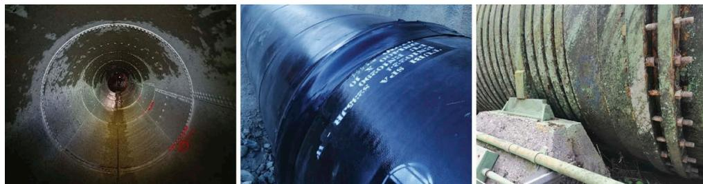
Figure 2. (a) Pipe with riveted joints; (b) Spiral-welded pipes with ball & socket joints; (c) Pipe reinforced on the outside with stiffener rings and expansion joint © Kager.
