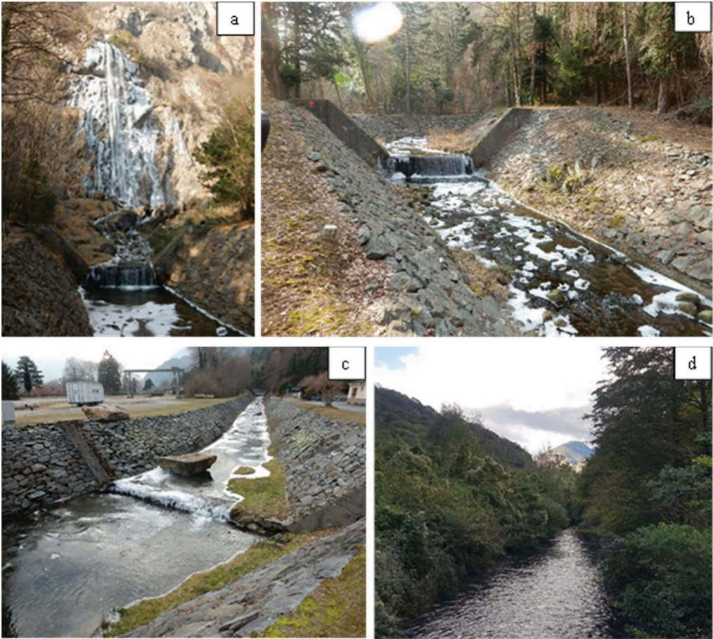
Figure 1. Photographs of the Salanfe River in the plain a) at the foot of the Cascade la Pissevache, with weir 1 in the foreground, b) on the channelled section at weir 2, c) then at weir 3, and d) in the Bois de Miéville.
