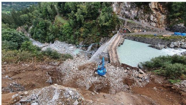
Figure 8. Overview of the excavation with the service gangway and the protection of the dam.
