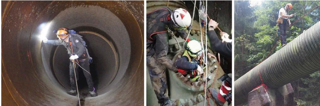
Figure 6. (a) Inspection activity inside; (b) Exit from a manhole; (c) Inspection activity outside with professional securing © Kager.
