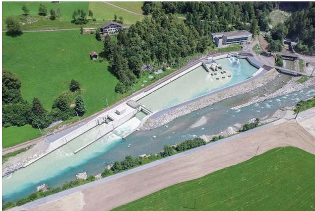
Figure 8. Innertkirchen hydropeaking compensation basin (Canton Berne) of Kraftwerke Oberhasli KWO (photo: KWO AG).
