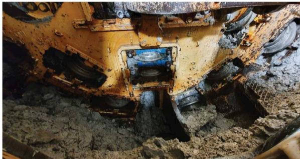
Figure 5. Cutter head at the fault gouge at tunnel meter 451.10.
