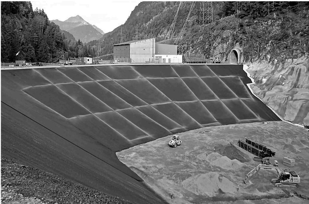
Figure 4. Layout of fiber-optic deformation measurement system.
