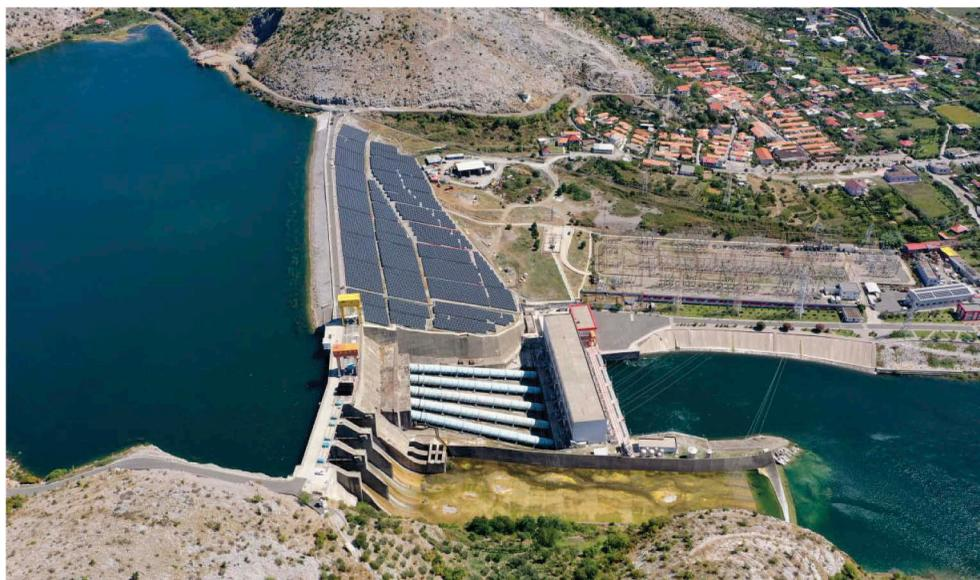
Figure 6. Photovoltaic plant on Qyrsaqi Dam of Vau i Dejes HPP.
