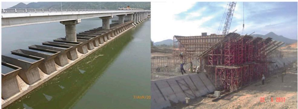
Figure 10. a) View of Van Phong dam barrage with the FSL, b) During construction.
