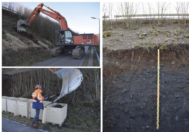
Figure 2. Sample collection for the triaxial tests.
