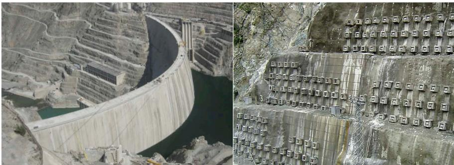
Figure 1. Upstream view of Deriner dam and rock stabilization of abutments.
