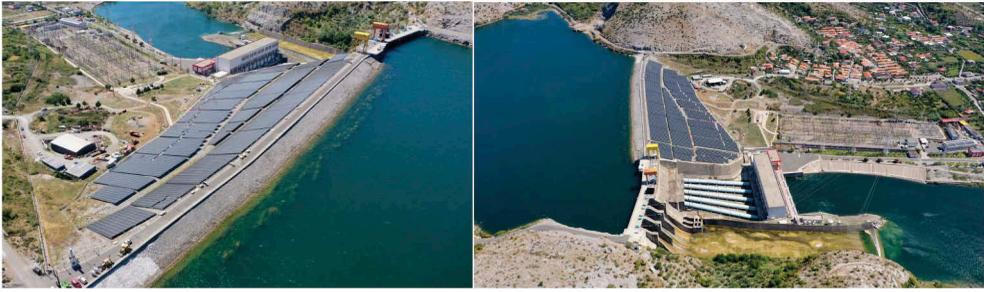
Figure 1. Views of PV Plant on the downstream face of Qyrsaqi Dam.
