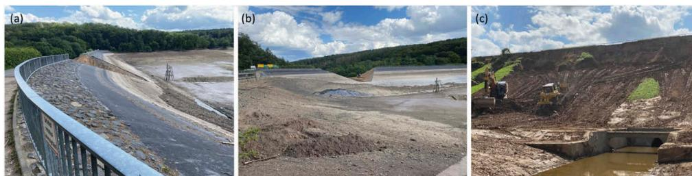
Figure 7. Steinbach Dam: (a) Dam crest, asphaltic membrane and embasure, (b) empty reservoir, (c) erosion gullies on landward dam side (all photos: Schüttrumpf).
