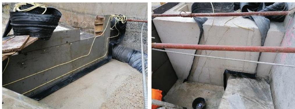
Figure 7. Details of the mass concrete block joints equipped with grouting compartments.
