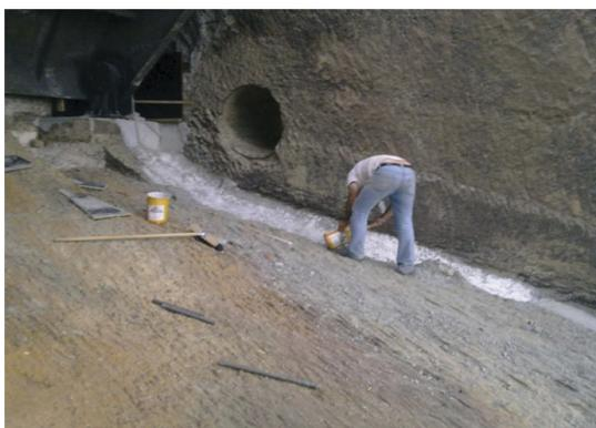
Figure 5. Application of epoxy binder.
