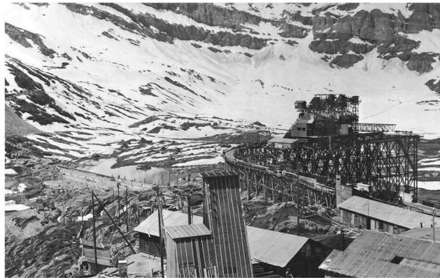
Figure 5. Salanfe dam. On the right, photo of the first stage dam, H=14.5 m.
