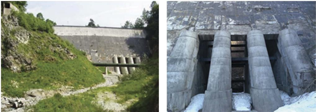
Figure 9. Combamala dam: opening at the bottom of the dam in 1997 (left). Particular of the opening in the structure (right).
