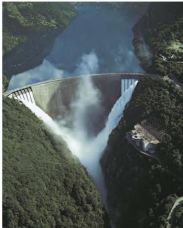
Figure 6. The Contra arch dam ( $H = 220$  m).
