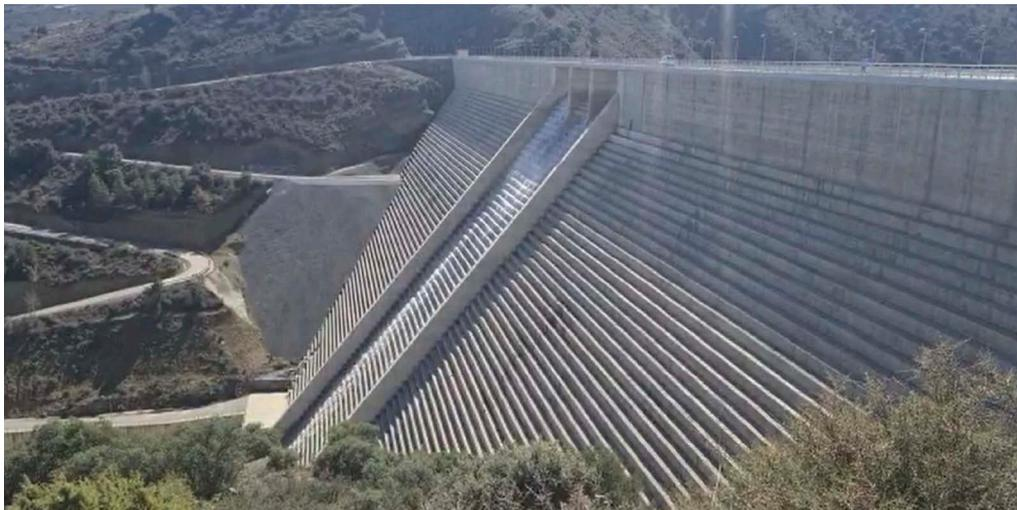
Figure 4. Enciso IV-RCC dam (105 m high). Downstream view during first spilling of the spillway.
