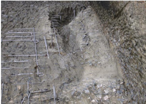
Figure 3. Spillway channel with damaged and pulled out surface steel reinforcements.
