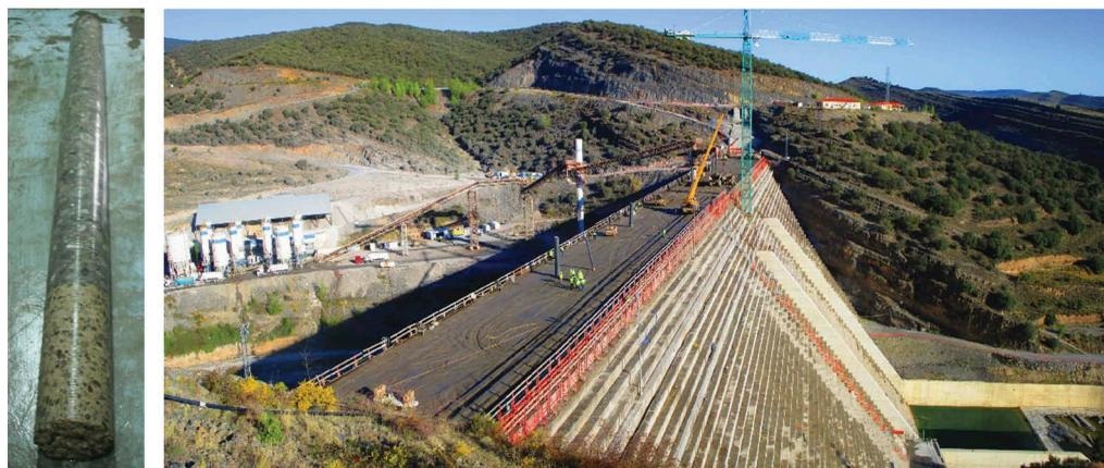
Figure 2. Vertical core of IV-RCC extracted from Enciso dam (Spain) and general view during construction.
