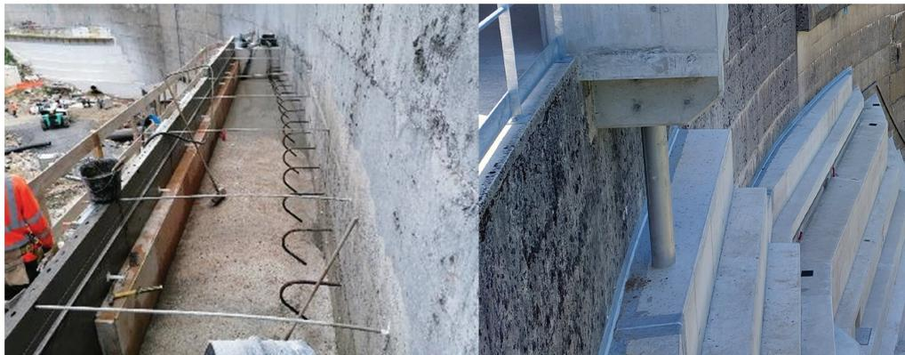
Figure 9. Bonding details: rebars during construction (left) and Hypalon band finish (right).
