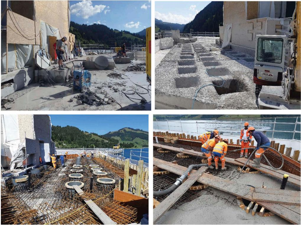
Figure 10. Concrete works. Top left, existing slab sawing and removal in pieces. Top right, hydro demolished surface of concrete ready to accommodate reinforcement and anchor heads. Bottom left, reinforcement being placed. Bottom right, concreting of new slab.
