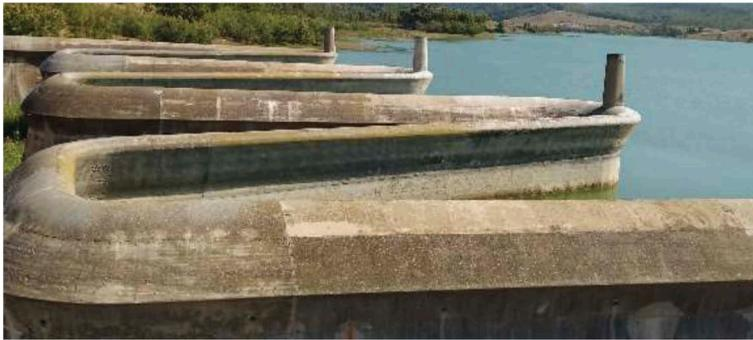
Figure 3. Labyrinth-type spillway.
