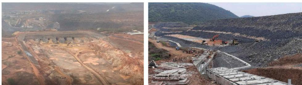
Figure 8. Pinnapuram pumped storage plant. At left, the rectangular upper reservoir under construction; in the background the intake structure of the penstocks leading to the downstream channel conveying water to the lower reservoir can be seen. At right, raising of one of the three dams forming the lower reservoir, with the plinth in the foreground.
