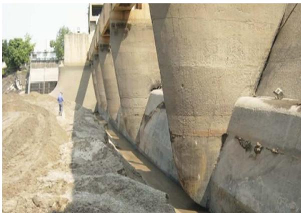
Figure 1. Sediments accumulated near the upstream face of the dam, after opening a 3 m high trench.
