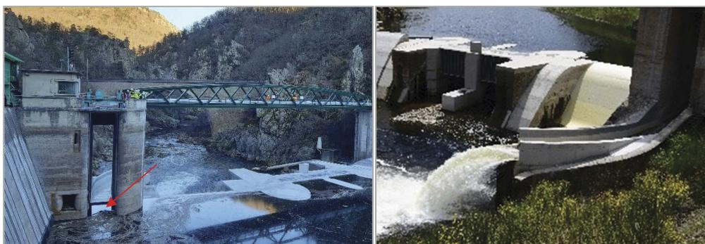
Figure 4. Reconfiguration of the downstream structure. Left, upstream view of the spillway (flap gate). Right, view of the downstream extremity of the spillway chute and the "spoon".
