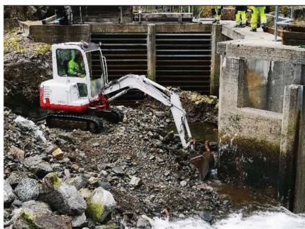
Figure 8. Conventional maintenance with excavator that has to be brought in by helicopter.
