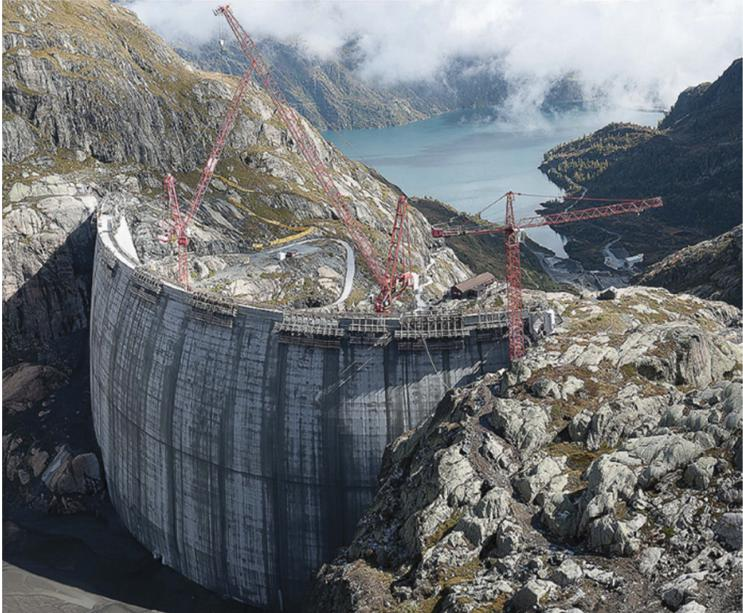
Figure 12. Nant de Drance PSP – heightening of the Vieux-Emosson dam – upper reservoir.
