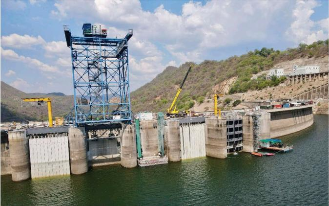
Figure 3. 40 m-high needles installed on two spillway sluices on Kariba dam (Zambia-Zimbabwe).
