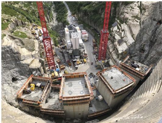
Figure 9. Spitallamm dam under construction in front of the existing arch-gravity dam (Courtesy A. Schleiss, 2022).
