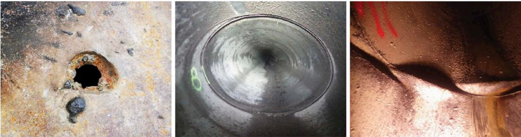
Figure 5. (a) Corrosion craters due to the action of stray currents; (b) Ovalization due to improper compaction of the pipe trench; Figure (c) Deformation in the area of an anchoring block © Kager.
