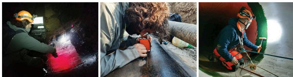
Figure 8. (a) Laser scan measurement in the pipe; (b) Analysis of the coating with P.I.G (Paint Inspection Gauge); (c) Checking the coating of a newly laid pipeline for pores © Kager.
