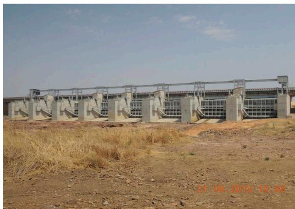
Figure 3. View of the 8 new radial gates.
