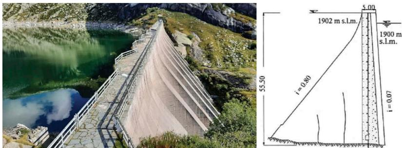
Figure 2. The Lago Eugio dam operated by IREN Energia in Piedmont (Italy), and the crack pattern in a buttress.
