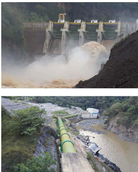
Figure 6. Jet trajectory and scour damage following 2017 flood (source: O. Jiménez).
