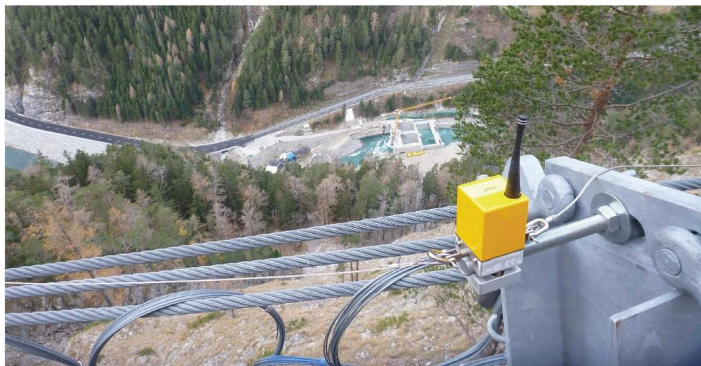
Figure 5. Rockfall barrier installed above the construction site close to Ovella, with one of the motion sensors installed to detect vibration and rockfall impact.
