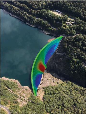
Figure 3. An automated numerical model for the assessment of the dam safety in real time.
