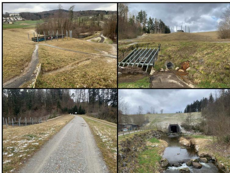
Figure 2. Jonenbach Dam upstream slope with spillway intake structure (top left), dam upstream slope with low-level outlet intake (top right), dam crest (bottom left), and dam downstream slope with combined outlet structure for spillway and low-level outlet (bottom right).
