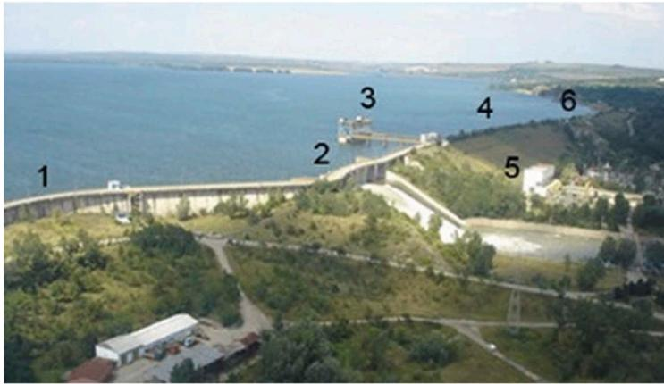
Figure 2. Aerial view of Stanca-Costesti dam. 1-Right wing dam; 2-Spillways; 3-Intake; 4-Main dam; 5-Powerhouse; 6-Old quarry closure dam.
