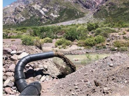
Figure 3. Discharge downstream of the dam crest. The discharge of sediments is controlled and corresponds to the capacity of the river.
