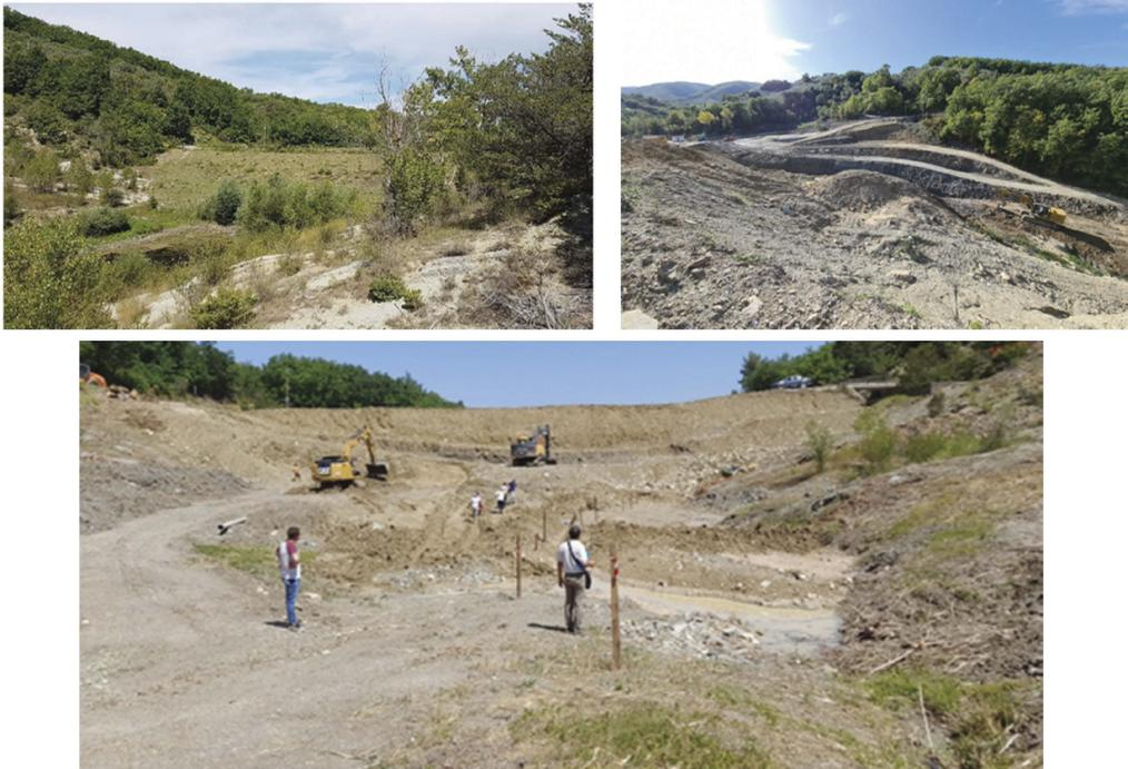
Figure 12. San Felice di Giano dam: the dam seen from upstream (up-left); reshaping of the riverbed and banks of the watercourse (up-right); the decommissioning works in progress (down).
