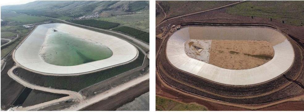
Figure 4. Kokhav Hayarden pumped storage plant. At left, start of impounding at lower reservoir, at right, waterproofing works completed at the upper reservoir.
