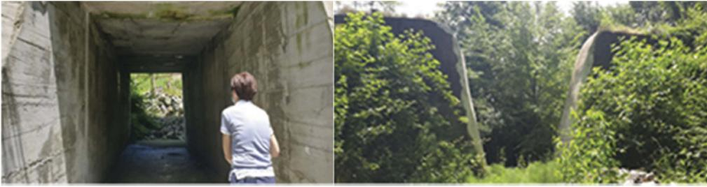
Figure 13. The gallery (left) and breach (right) opened respectively in the main and small Galano dams in 2019.
