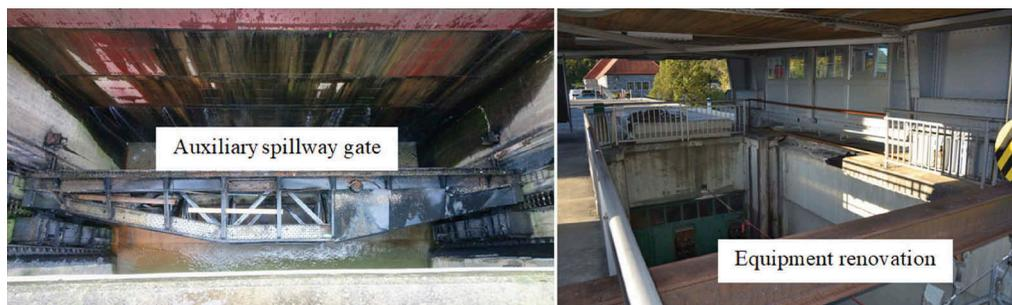
Figure 8. Rehabilitation works on the Mariborski otok Dam.
