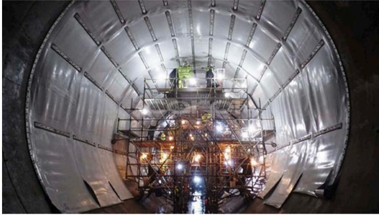
Figure 2. Application of an exposed geomembrane system in pressure waterways; illustration of the Helms penstock access tunnel, USA; geomembrane system with fastening system and perimeter seals. Image: courtesy of Carpi Tech.
