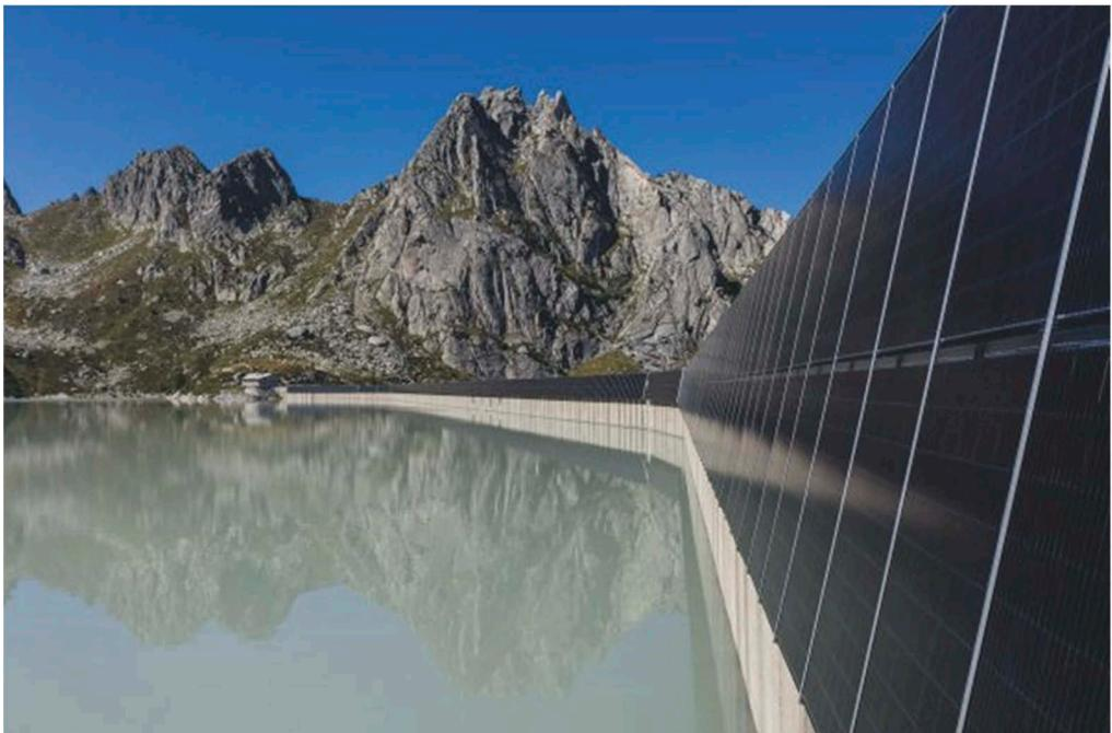
Figure 3. DMPV plant on the Albigna dam (© ewz).
