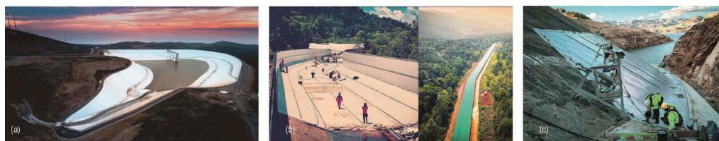
Figure 1. Examples of GS applications in hydropower: (a) reservoir of Pico da Urze pumped storage plant, Portugal, (b) hydraulic canal of Larona hydropower plant, Indonesia, (c) upstream pumped face of Paradelada dam, Portugal. Images: courtesy of Carpitech.
