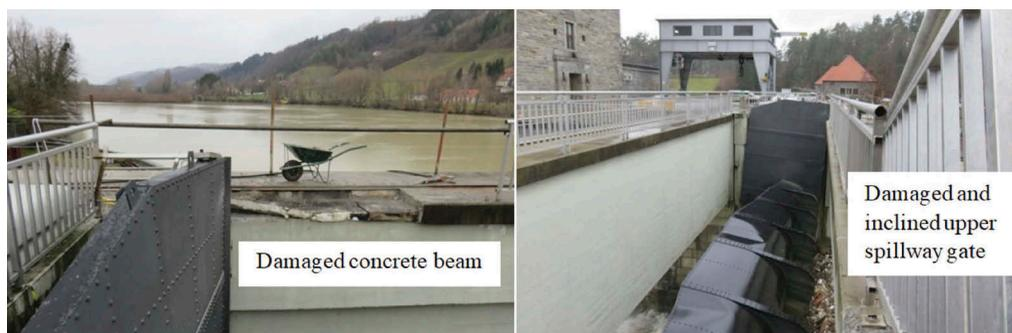
Figure 7. Damaged concrete beam and damaged upper spillway gate on the Mariborski otok Dam.
