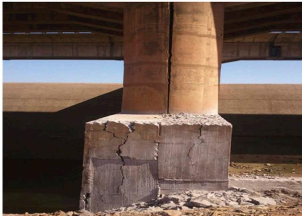
Figure 1. Longitudinal joints of the abutments.
