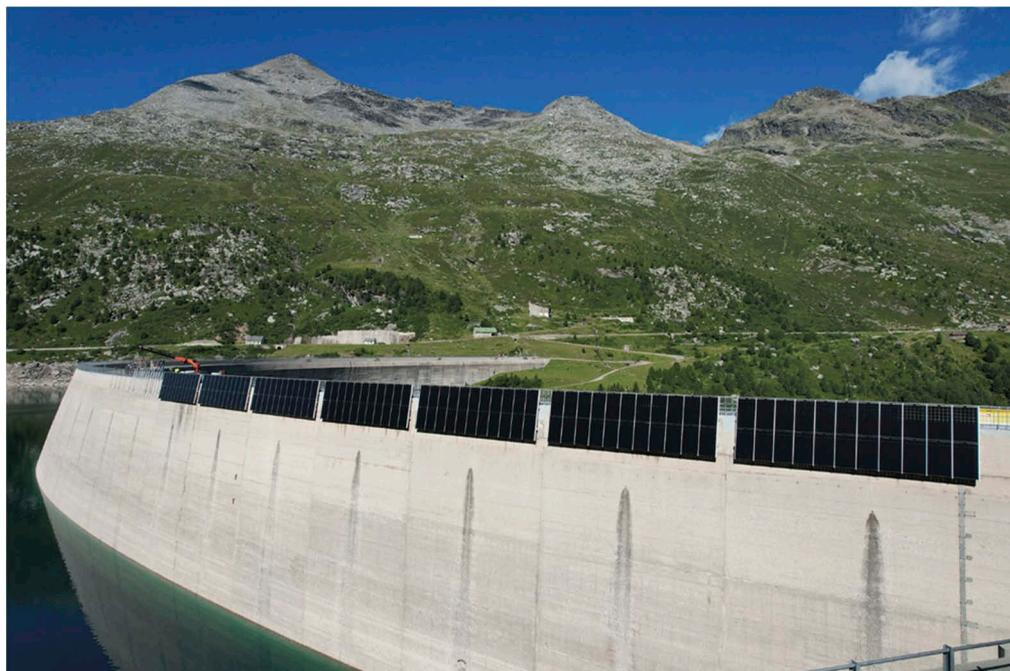
Figure 4. DMPV plant on the Valle di Lei dam (© ewz).
