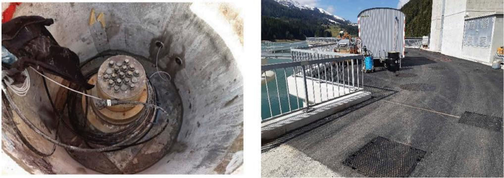
Figure 12. Left, strands excess length cutting. Right, final state of the artificial gravity abutment.
