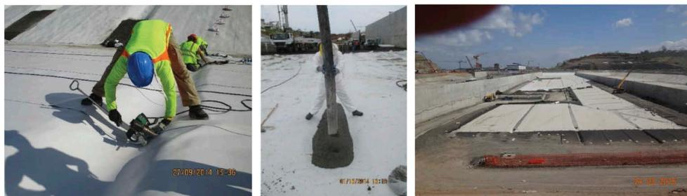
Figure 1. Panama Canal Expansion Water Saving Basins. Anchorage by tensioning trenches on the invert. These trenches avoid the formation of loose areas and folds in the geomembrane, which is crucial in these basins with several daily water level fluctuations, and thus ensure the longevity of the system.
