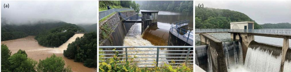
Figure 5. Overflow of spillways: (a) Urft Dam, (b) Perlenbach Dam, (c) Rur Dam (photos: (a) and (c) Vonden, (b) Schüttrumpf).
