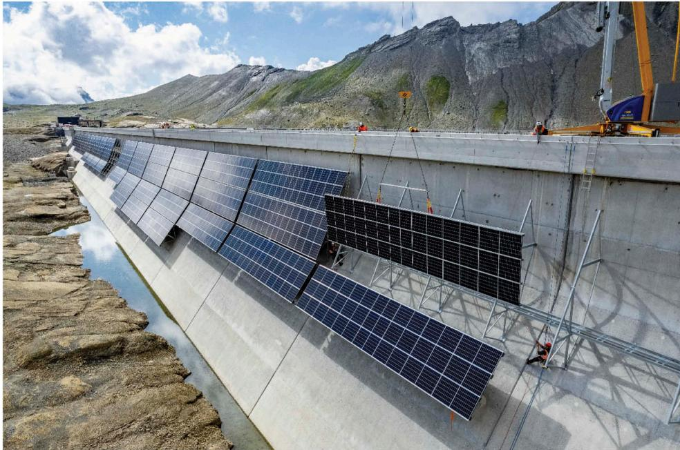
Figure 3. Construction phase of the PV system on the Muttssee dam<sup>2</sup>.
