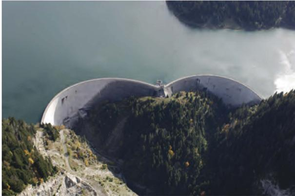
Figure 5. The double-arch Hongrin dam ( $H = 125/90$  m).
