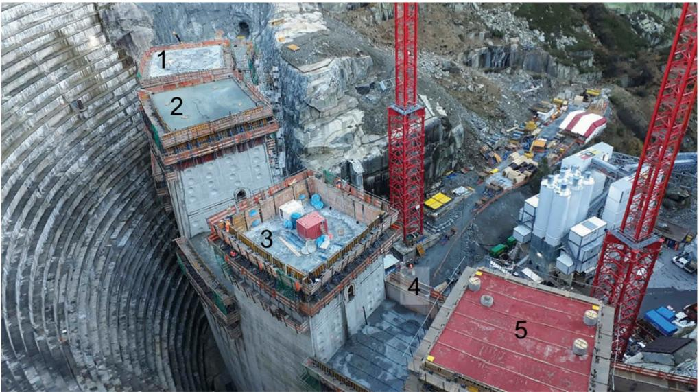
Figure 5. Leader and follower blocks at different stages (25.10.2022). From left to right: (1) hard concrete after green cut, (2) fresh concrete, (3) formwork recently lifted with shear keys being placed, (4) lift cleaned and ready for casting with cooling pipes, and (5) lift covered with thermal cover, ready for the Winter break.
