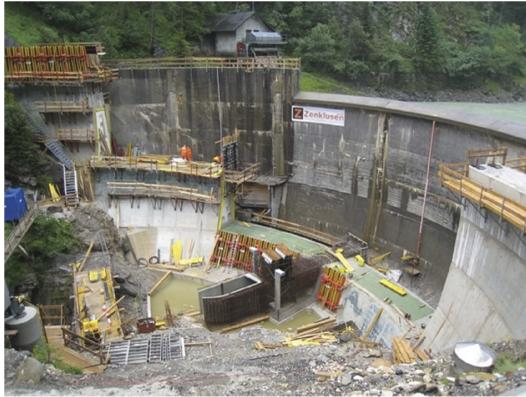
Figure 8. Serra Dam during reconstruction: new arch dam in front of the old dam before its partial demolishing.
