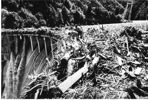
Figure 10. Blocked passes at the Palagnedra dam (TI) during the flood on August 7, 1978.
