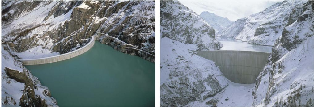
Figure 3. The Mauvoisin arch dam (H = 250 m).
