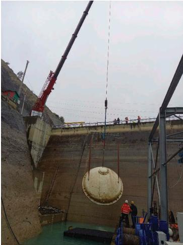
Figure 1. Left: Removal of the 4 m-obturator on Idriss I dam (Morocco).
