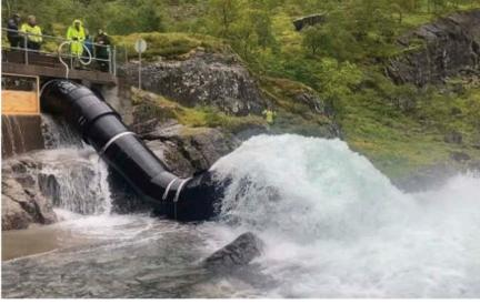
Figure 10. Boulder excluder during operation in September 2022.
