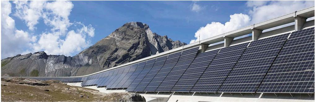
Figure 2. DMPV plant on the Muttssee dam (© AlpinSolar).
