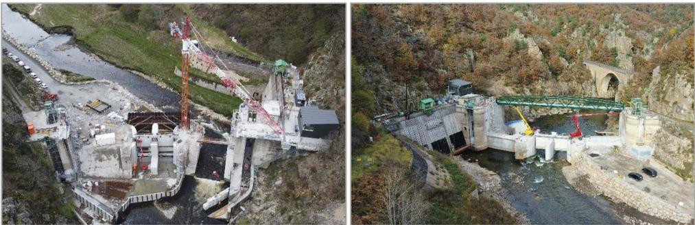
Figure 9. Aerial views of the dam reconfiguration during the construction phase.
