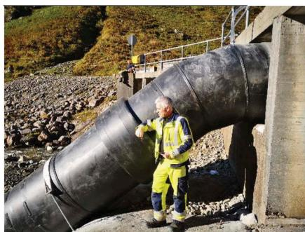
Figure 9. Boulder excluder after installation.
