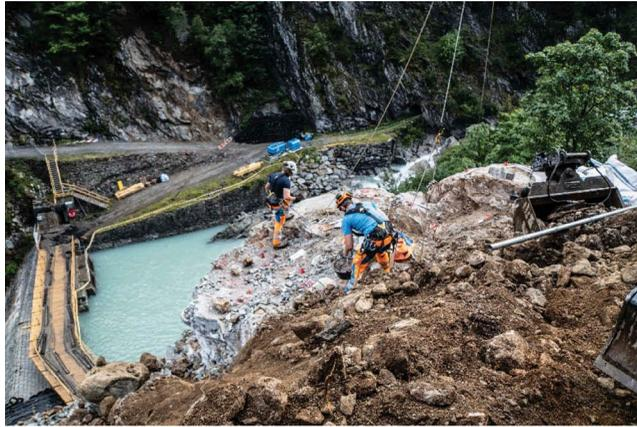
Figure 7. Loading the blast holes, excavation of approx. 100 m<sup>3</sup> of materials.
