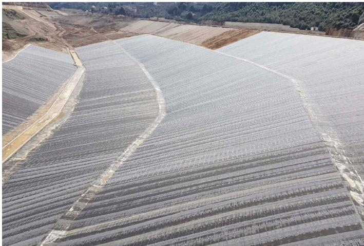
Figure 9. Example of a reservoir slope reshaping and a geomembrane lining installation for preventing water leakage in karst and fissured rock formations (Middle East).
