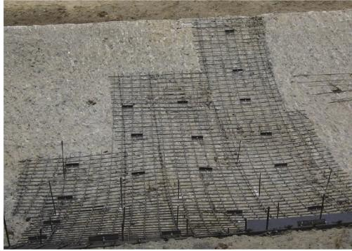
Figure 7. Repair of the spillway channel surface.
