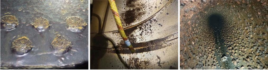
Figure 4. (a) Abrasion phenomena at riveted joints close to the ground; (b) Abrasion phenomena in the area of a slope change; (c) Corrosion due to unsuitable coating © Kager.
