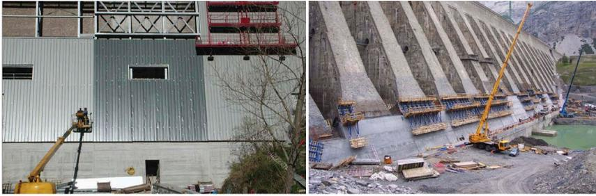
Figure 4. The steel insulating shield built to cover the buttresses of Ancipa dam (left), operated by ENEL Green Power in Sicily (Italy), and the weighting of San Giacomo di Fraele dam (right), operated by A2A in Lombardy (Italy).
