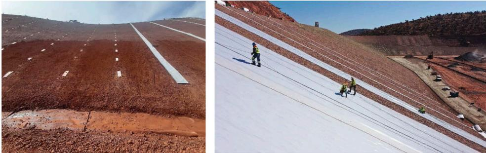
Figure 6. Abdelmoumen pumped storage plant. At left, the geomembrane anchor wings embedded in the embankment, and the geomembrane anchor band heat-seamed unto the wings. At right, the geomembrane liner under installation on the slopes.
