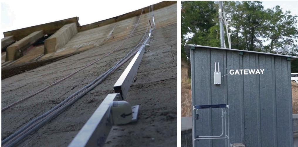
Figure 2. Wireless sensor array (left) and the associated wireless gateway (right).
