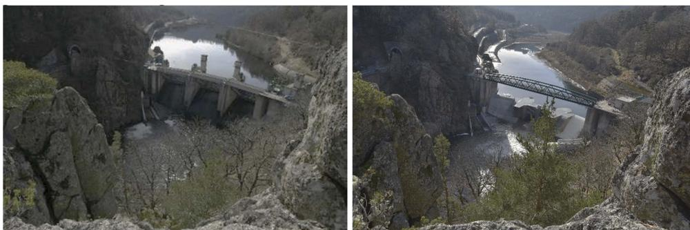
Figure 5. Retrofitting of the Poutès dam. On the left, before works. On the right, after works.
