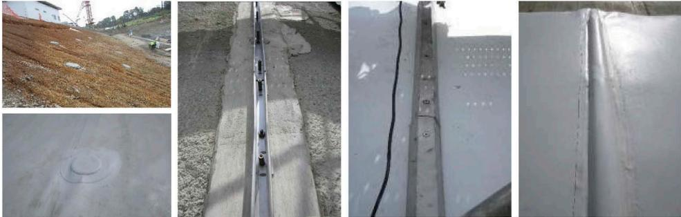
Figure 2. Panama Canal Expansion Water Saving Basins. Anchorage at points (at left) and by with tensioning profiles secured with deep anchors or chemical anchors, depending on the conditions of the subgrade.
