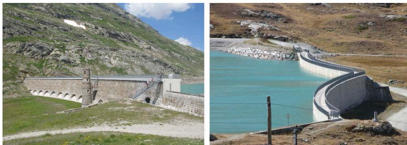
Figure 2. Scala arch-gravity dam with overflow section (left) and Arlas gravity dam (right).
