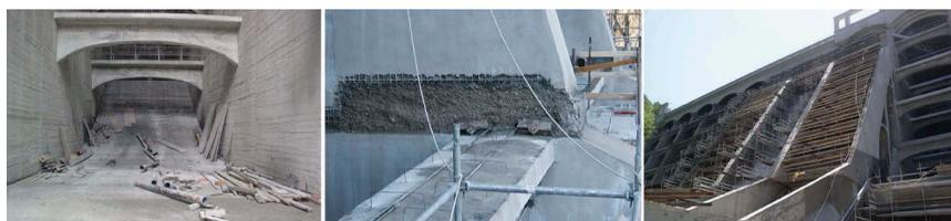
Figure 8. Weighting of the dam foundation (left), strengthening of T-shaped beams with tie rods (center) rehabilitation of the surface spillway.
