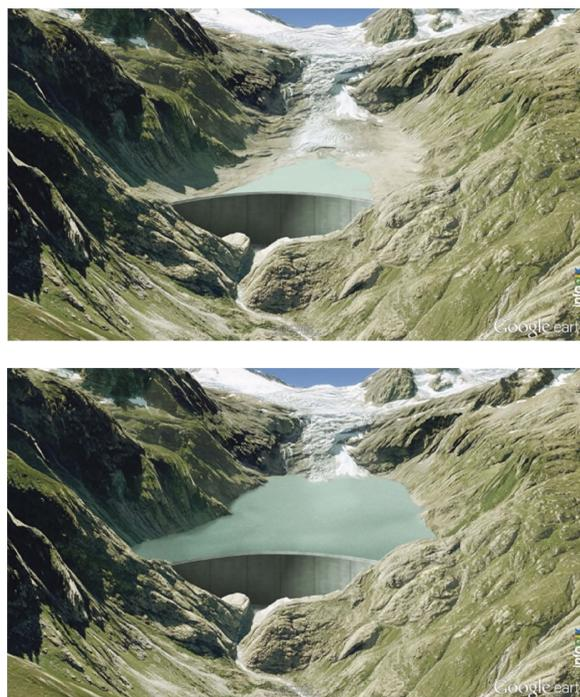
Figure 11. Photomontage of the future 180 m high Trift dam, which uses the already freed valley by glacier retreat. Above: with empty lake with glacier position today. Below: with full lake (Curtesy KWO).
