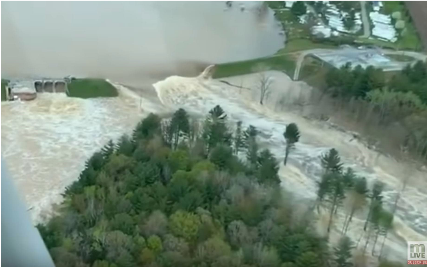
USA, Michigan - Edenville Dam 19. Mai 2020
