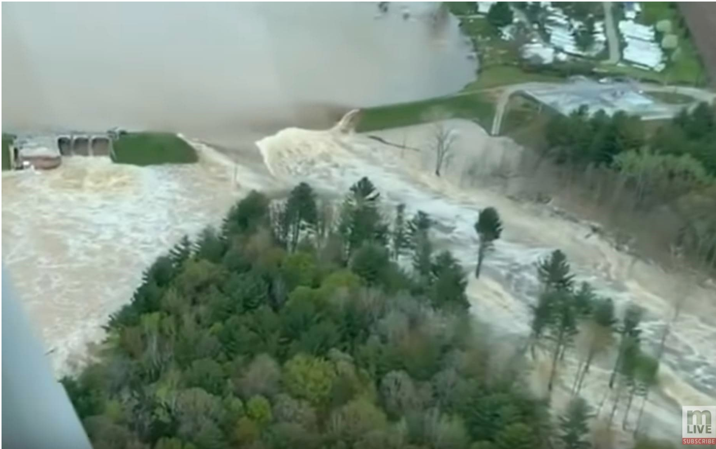
USA, Michigan - Edenville Dam 19. Mai 2020
